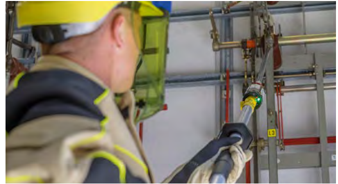
PHE III voltage detector with visual and acoustic indicator used for an indoor switchgear installation
