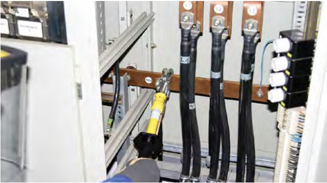
Attaching an earthing and short-circuiting device in a low-voltage switchgear installation using an earthing handle.
