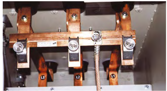
Short-circuiting bar with earthing cable on a switchgear installation.
