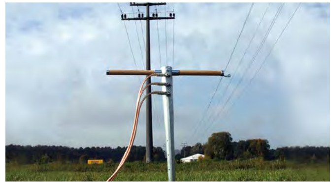
Earthing busbar and earthing cables mounted on a tubular earth electrode
