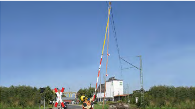
Attaching a railway earthing device.
