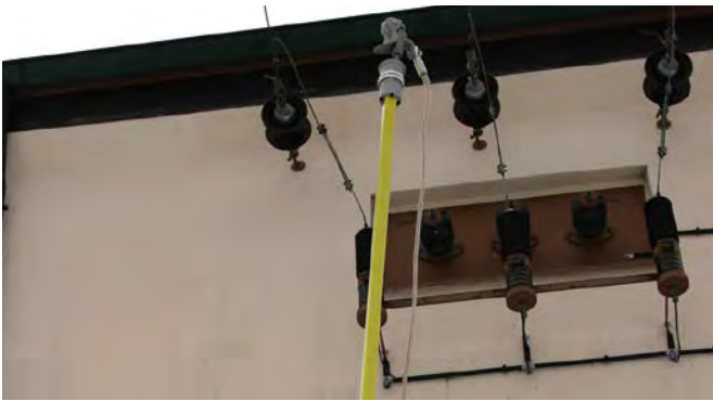
Telescopic earthing stick with aluminium cone coupling and phase screw clamp.
