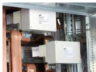
Quenching device above the supply switch
