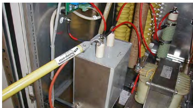
Single-pole device for discharging static charges
