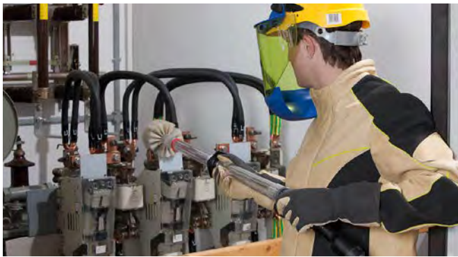
Live cleaning of a transformer using the TRS MS dry cleaning kit.
