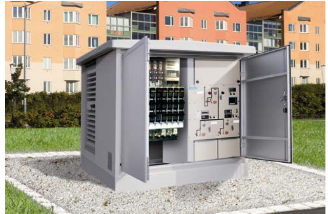
Postes de distribution intelligents
