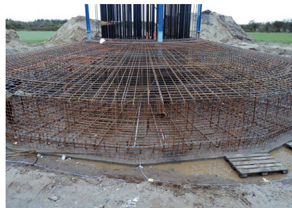
Figure 3 Reinforcement of a wind turbine with foundation earth electrode
