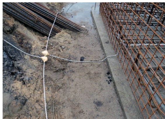
Figure 7 Ring earth electrode connected to the foundation earth electrode
