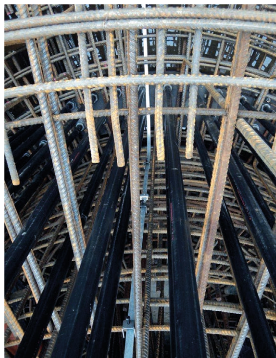
Figure 6 Connection of the earth electrode to the reinforcement
