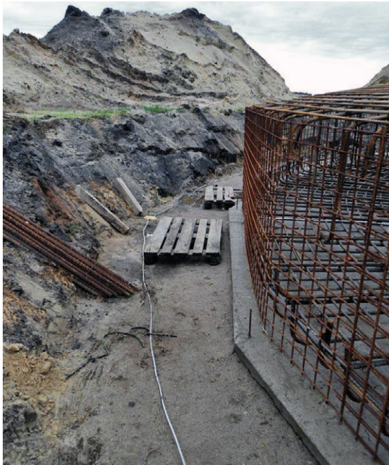
Figure 8 Reinforcement of a wind turbine with buried ring earth electrode
