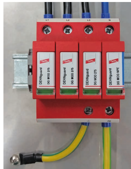
Figure 9 Additional local equipotential bonding, e.g. via the metal enclosure/mounting plate of the switchgear installation
