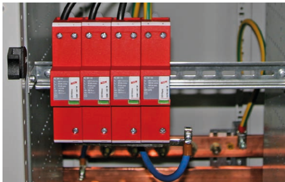
Figure 8 Coordinated type 1 surge arrester
