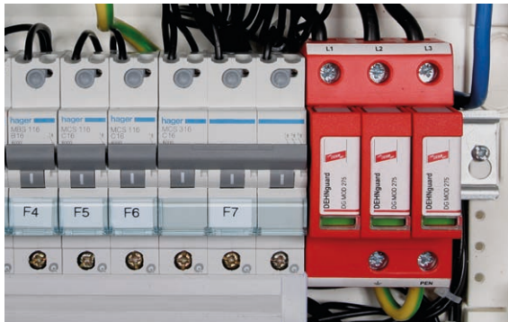
Figure 6 Modular type 2 surge arrester for protecting the 230/400 V supply
